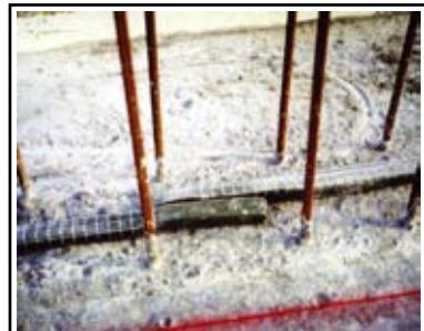
**• field of application** | Secure installation of Bentorub®+ in horizontal and vertical applications.
